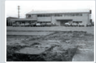
Construction of Hiroishi Plant
