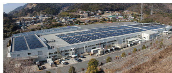
Solar panel of Osawa Plant
